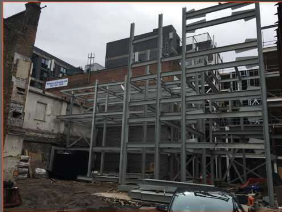
Part erection of steel frames currently on site
